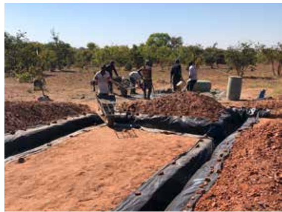
The foundation was being dug
